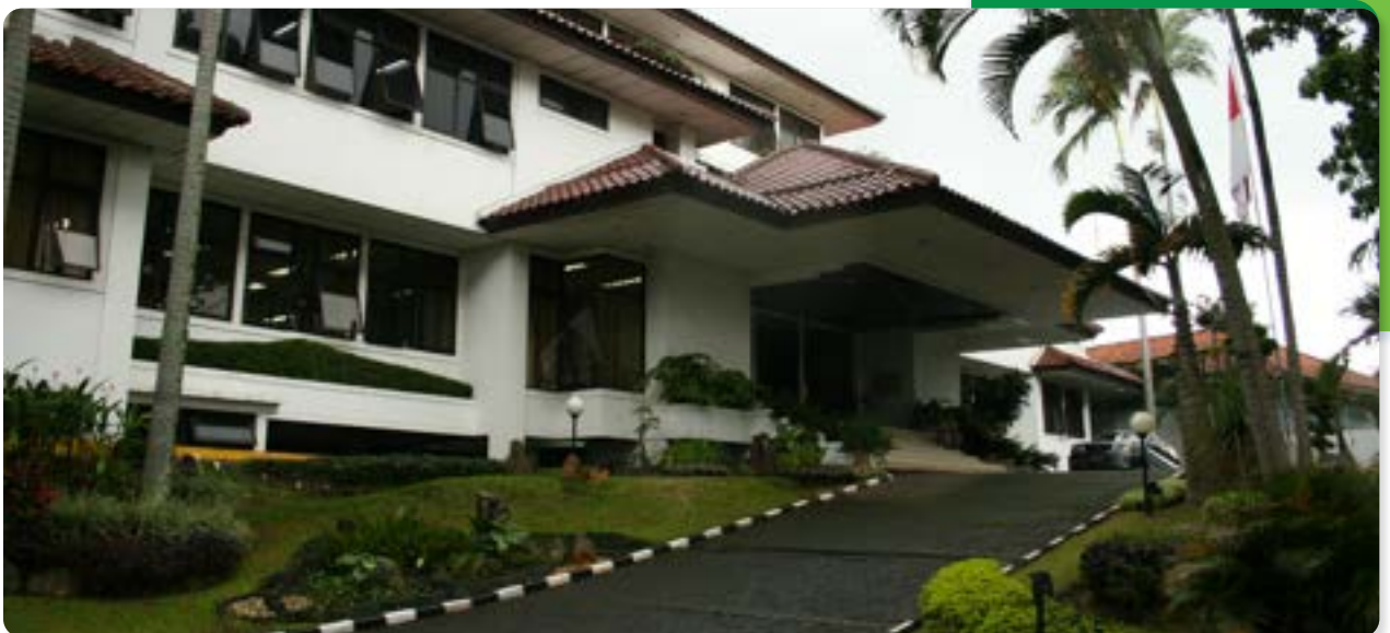
Fasilitas Kantor Regional 2 Regional Office 2 Facilities
