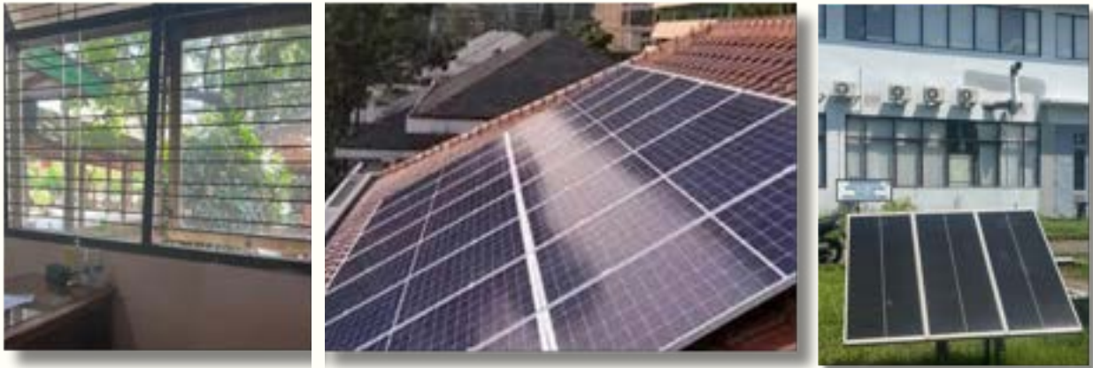
Figure 35. Image of a building with ventilation and solar panels
