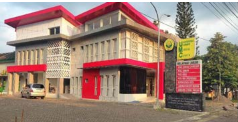
Figure 72. RSGM and UMC Building
