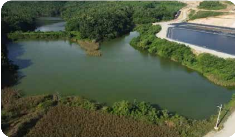
▲ BSI's dam 5 and 6 to collect raw water and precipitate sediment in rainwater
