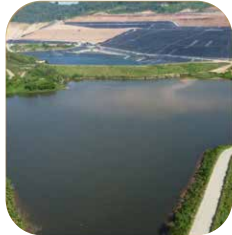
▲ BSI's dam 4 to collect rainwater from heapleach area
