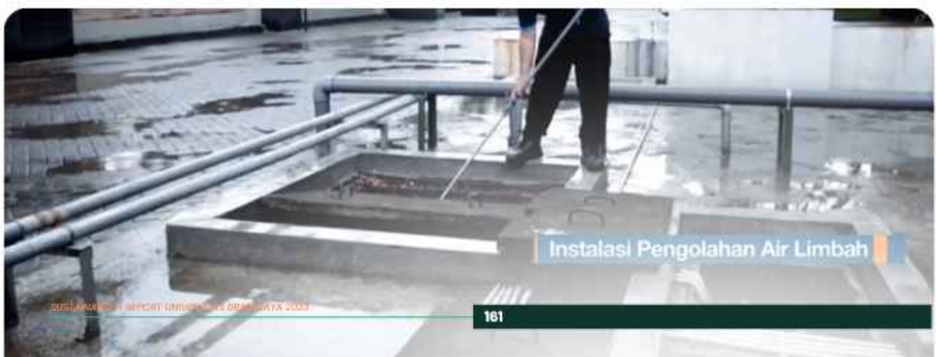
Instalasi Pengolahan Air Limbah UB UB Wastewater Treatment Plant (IPAL)
