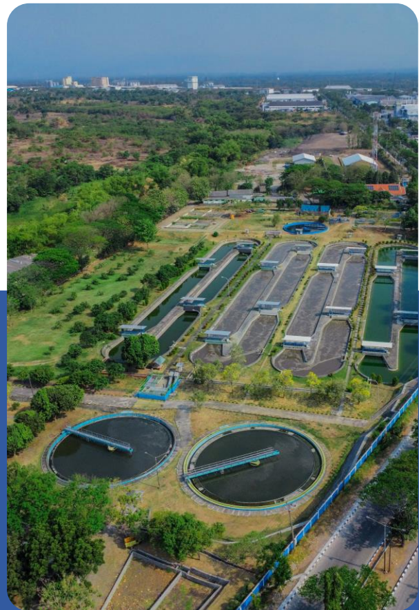
TPST 3R (Pengelolaan Sampah Industri) TPST 3R (Industrial Waste Management)
