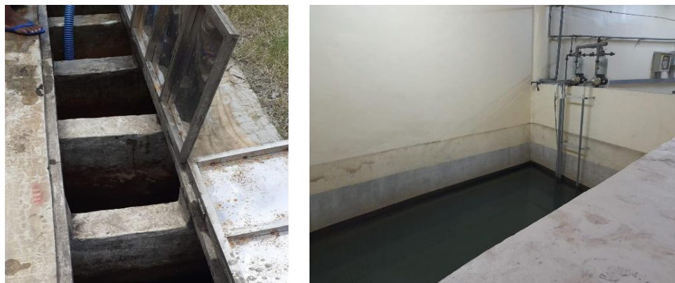
Gambar 97. IPAL Kantin dan Tampungan Air Sisa Wudhu di Universitas Jember Figure 97. Canteen IPAL and Ablution Wastewater Reservoir at Jember University
