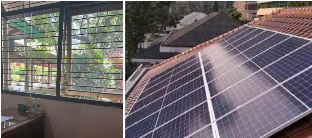
Gambar 75. Gambar Gedung Dengan Fentilasi Dan Panel Surya Figure 75. Image of a building with ventilation and solar panels
